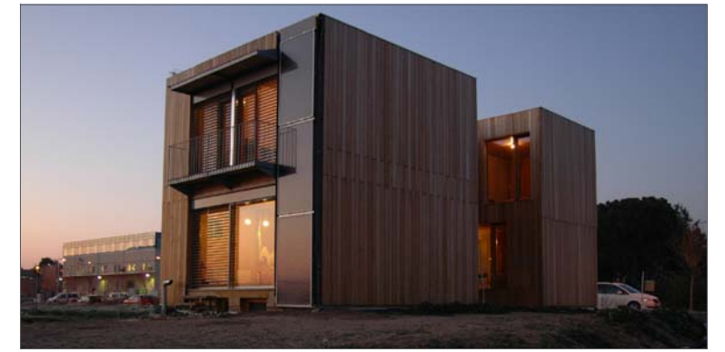
VISTA GENERAL_GENERAL VIEW
